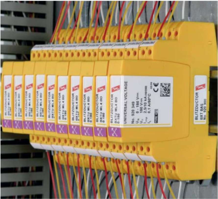
Figure 6.8.6(h) – Surge protection device for twisted pair cables (Dehn)
