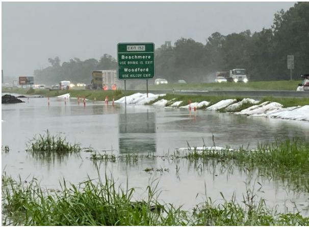
The result of over 100mm of rain at the site on Monday 22 March 2021.
