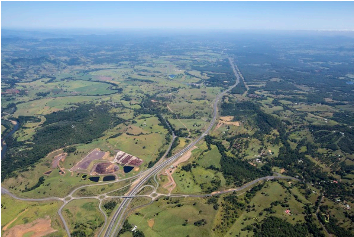
Figure 2 Completed Highway - Traveston Interchange north to Woondum
