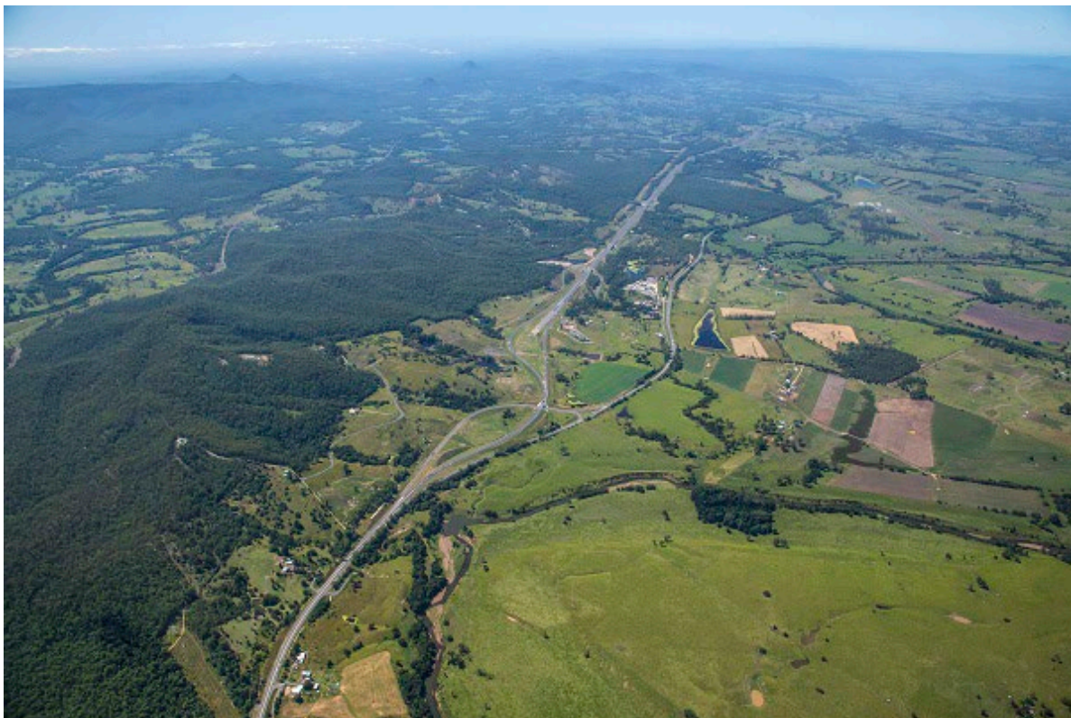
Figure 3 Completed Highway - Looking north to Woondum Interchange
