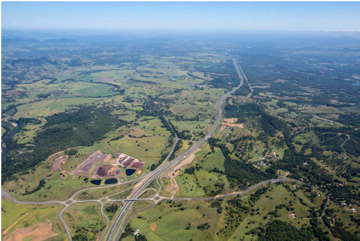
Figure 2 Completed Highway - Traveston Interchange north to Woondum
