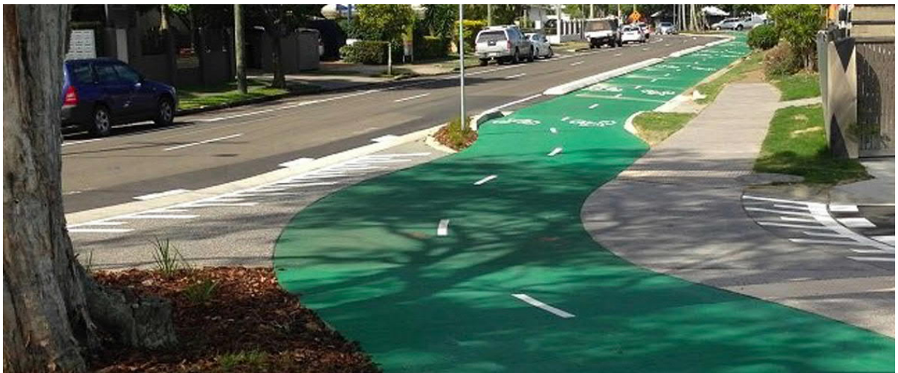
Figure 7-7: Example of a two way cycleway with driveways and side road crossings on a residential street (River Esplanade, Mooloolaba)
