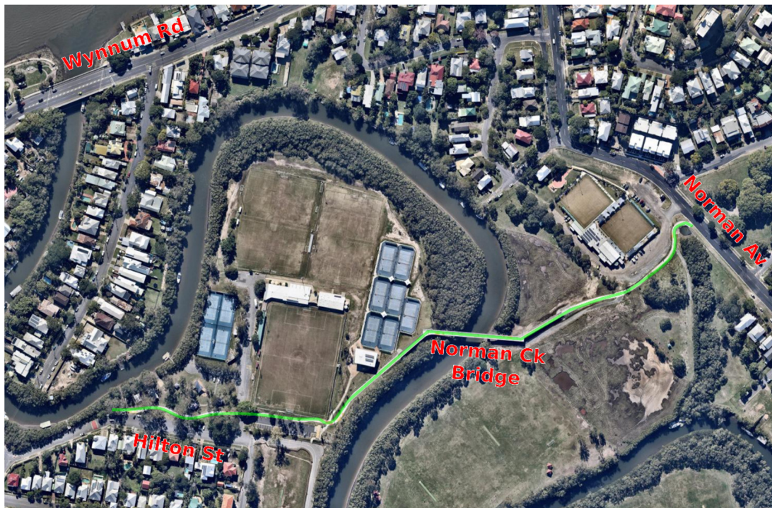
■ Figure 1.1: Norman Creek Bridge (aerial image: Nearmap, 1 Jul 2016)
