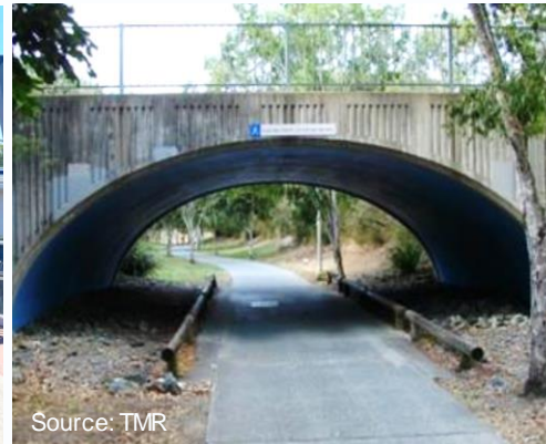
Wide CPTED underpass
