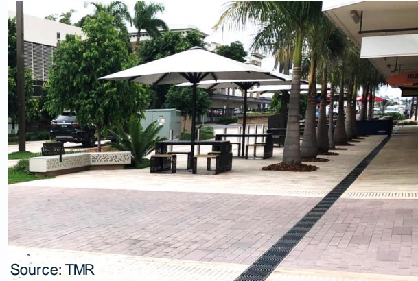
Integrated drainage and shade
